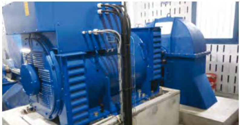
L'Aya hydroelectric power station
