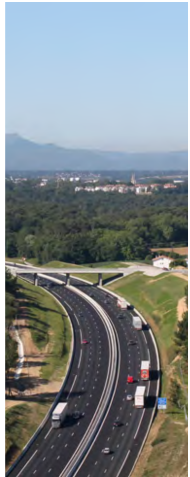
Widening the A63 between Ondres and Saint-Geours-de-Maremne (Aquitaine) to three lanes in both directions
