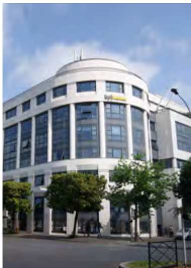
Bpifrance headquarters in Maisons-Alfort (Val-de-Marne)
